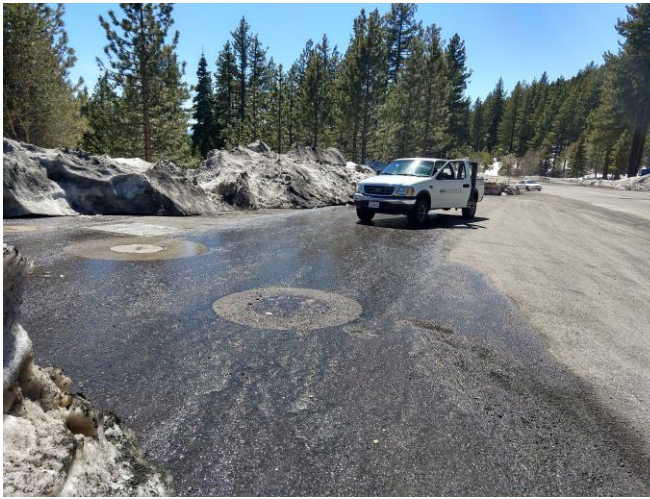
Figure 3: April 18, 2019 berm on pullout and road. Access doors are under berm.
