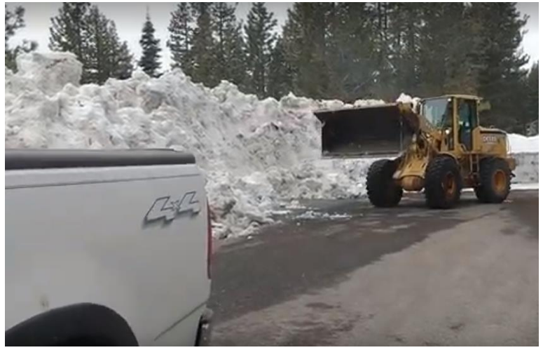
Figure 4: March 22, 2019 berm on pullout and road. Loader is removing snow to clear access doors under berm.
