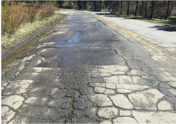
Figure 67 Elks Club Drive prior to repaving. (R Wigart)
