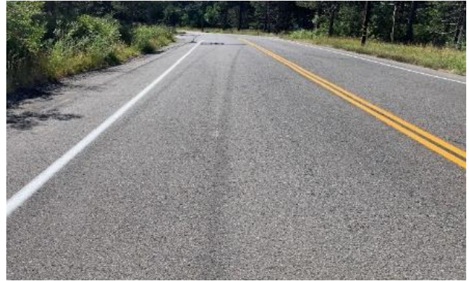
Figure 68 Elks Club Drive after repaving. (A Buxton)
