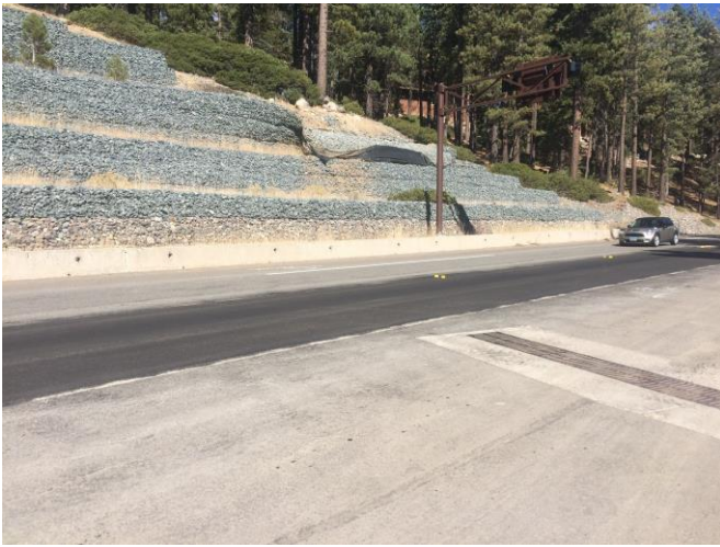
Figure 1: October 19, 2017 sediment on pullout and road.
