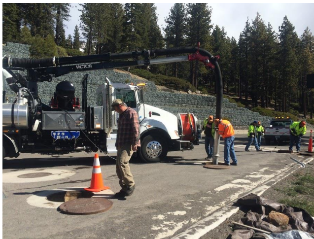
Vactor truck cleanout on 4/15/16 at SR431 (left). Note accumulated sediment along the curb. Sediment filled flume prior to cleanout (right).
