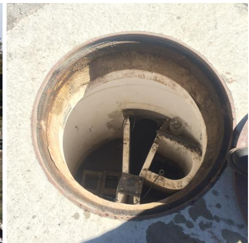
Vactor truck cleanout on 4/15/16 at SR431 (left). Note accumulated sediment along the curb. Sediment filled flume prior to cleanout (right).
