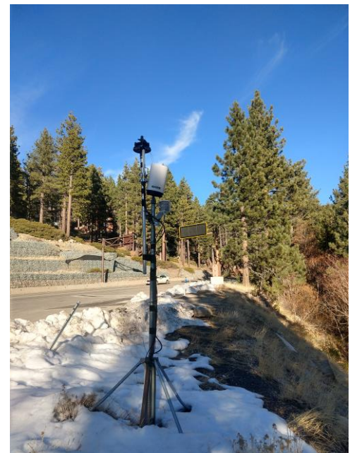
Figure 3: Tipping bucket damaged by snow removal efforts. Photo: December 3, 2020.
