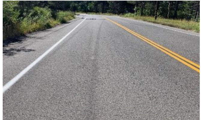
Figure 3 Elks Club Drive after repaving. (A Buxton)
