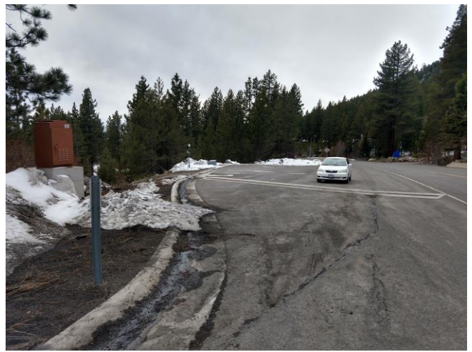
Figure 4 Snow berm and pullout SR431 on January 27, 2022.
