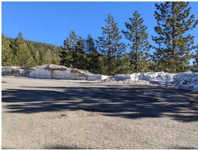
Figure 1 Snow berm on SR431 on January 27, 2022.
