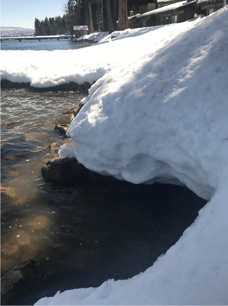
Figure 71 Backwatered conditions at the Tahoma catchment outfall due to high lake levels, March 23, 2018. The pipe is under the snow and the lake water extends into the flume.
