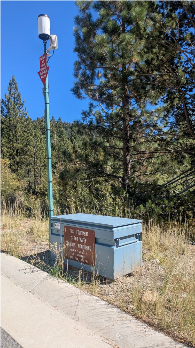
Figure 3 Equipment housing and meteorological station in excellent condition on 9/24/25.
