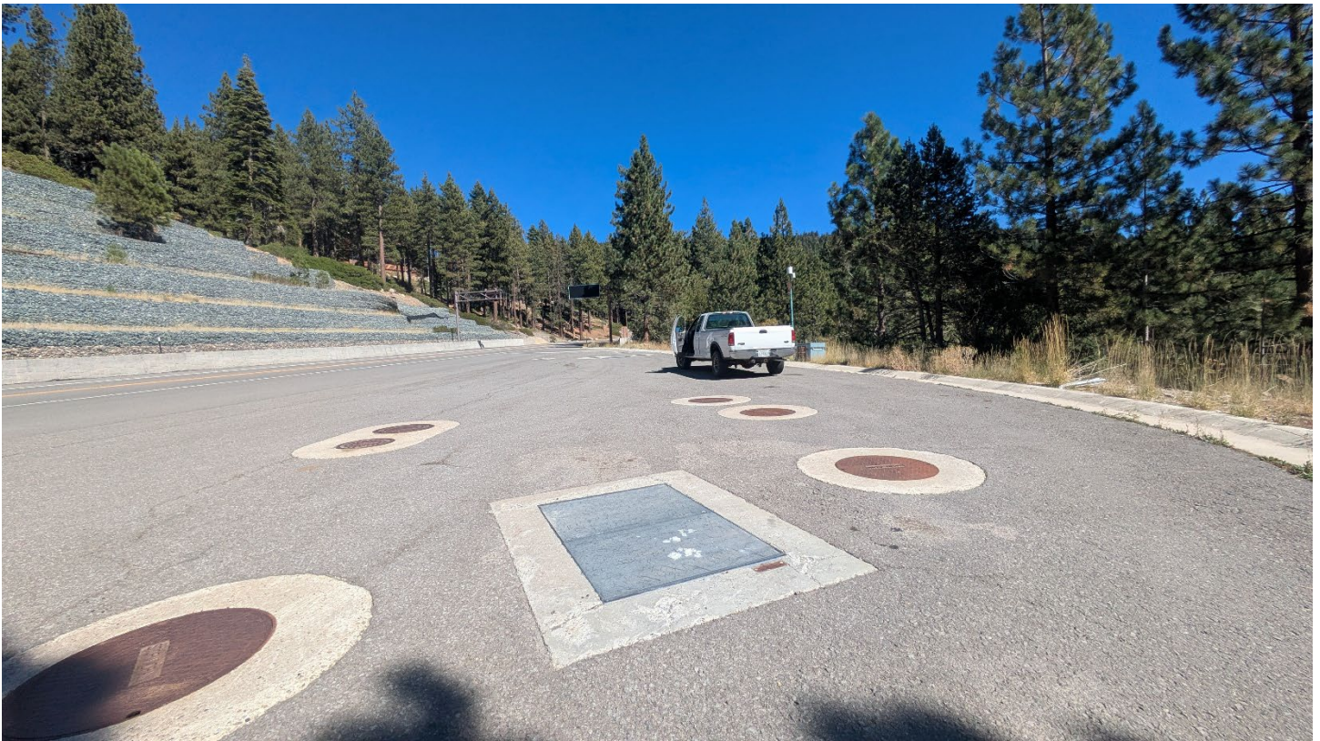
Figure 4 Pavement free of excessive sediment accumulation on 9/24/25.
